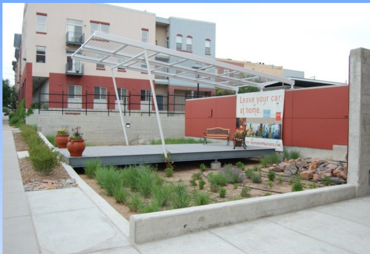
Rain Garden (Bioretention)
